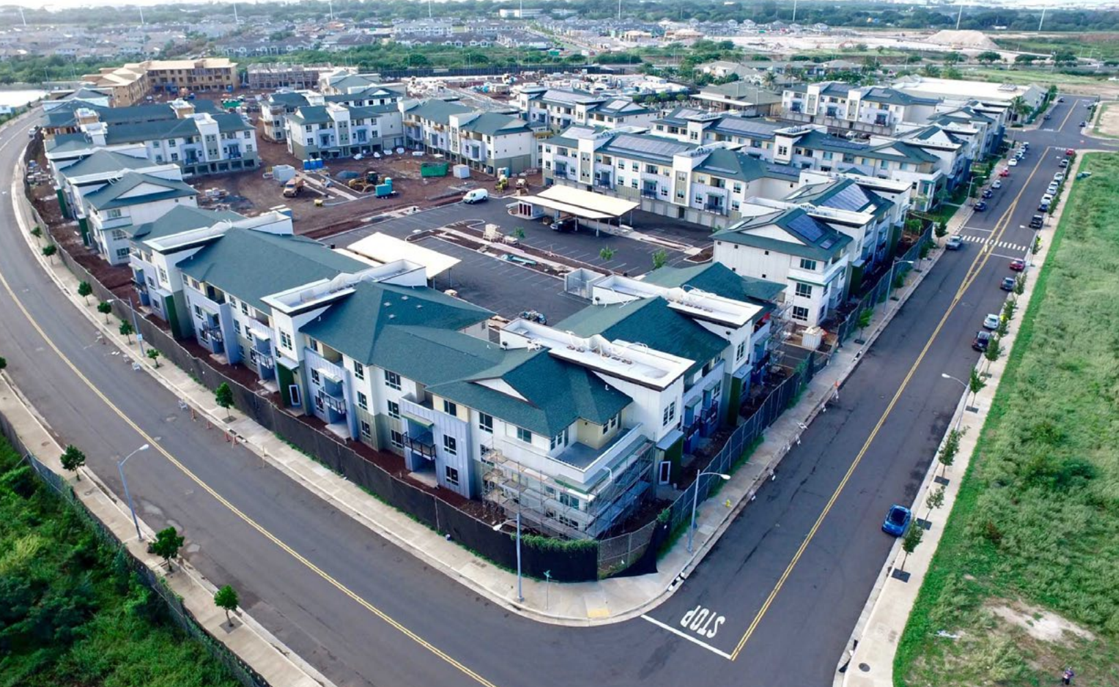
Steffes GETS system in a new development called Kapolei Lofts that will include 499 rental homes in western Oahu.
